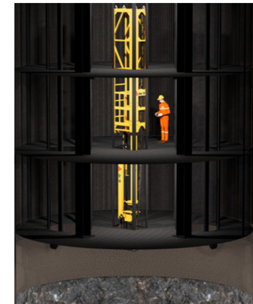
Safe position in the galloway during blasting
