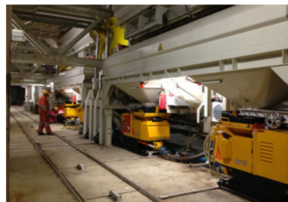
Pea gravel backfilling installation on TBM
